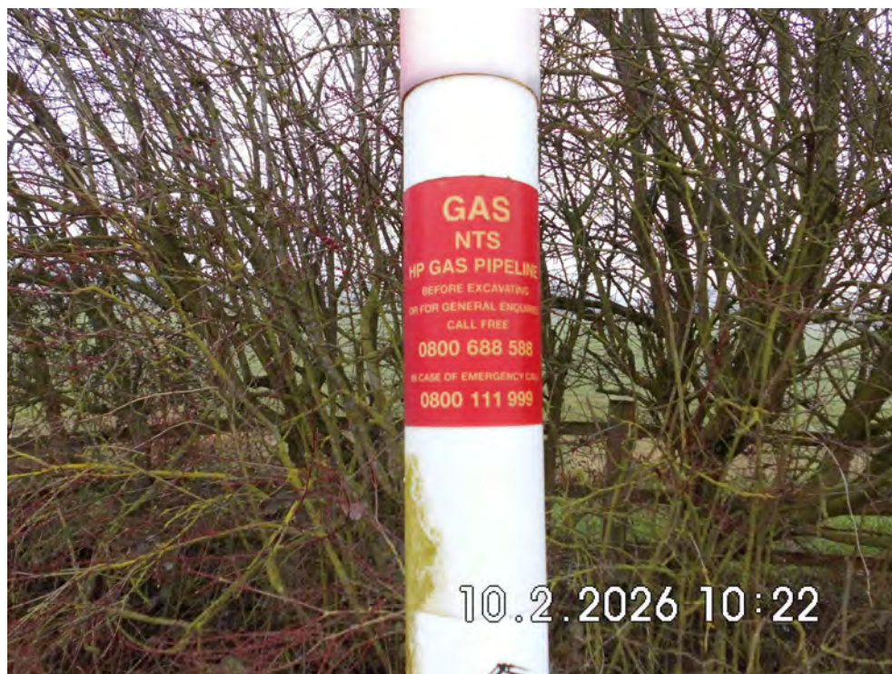
Fig 18.3 Photo of National Gas Transmission High Pressure Feeder No. 5 Marker pole within Site 5
