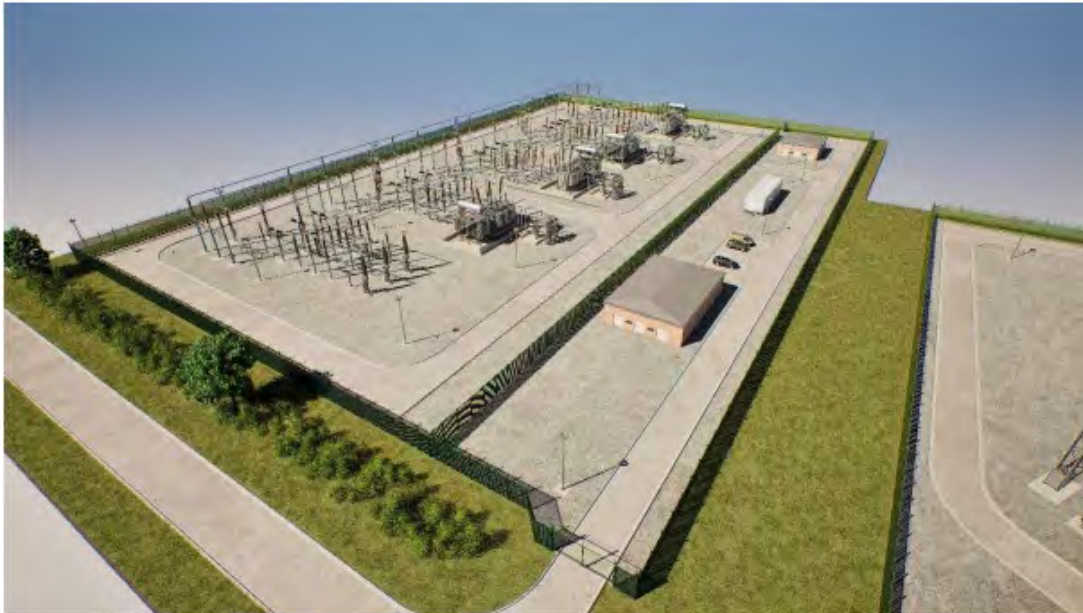
Figure 4.3 Environmental Statement Image 4.10 (Illustrative Air Insulated 400kV Substation)
