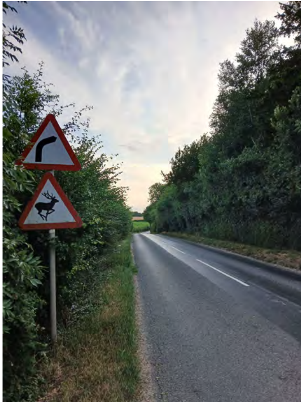
Figure 11.12 Photo of View looking along Northern Boundary of Site 5 towards Boylandhall Lane showing where the B1527 dips and then rises meaning forward visibility is obscured by the road surface. Also showing the Wild Animal Warning Road Sign
