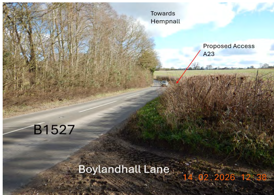
Figure 11.4 Photo of A23 Proposed Access point into Site 5
