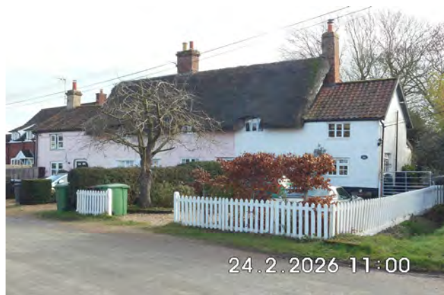
Wayside Cottages, The Street
