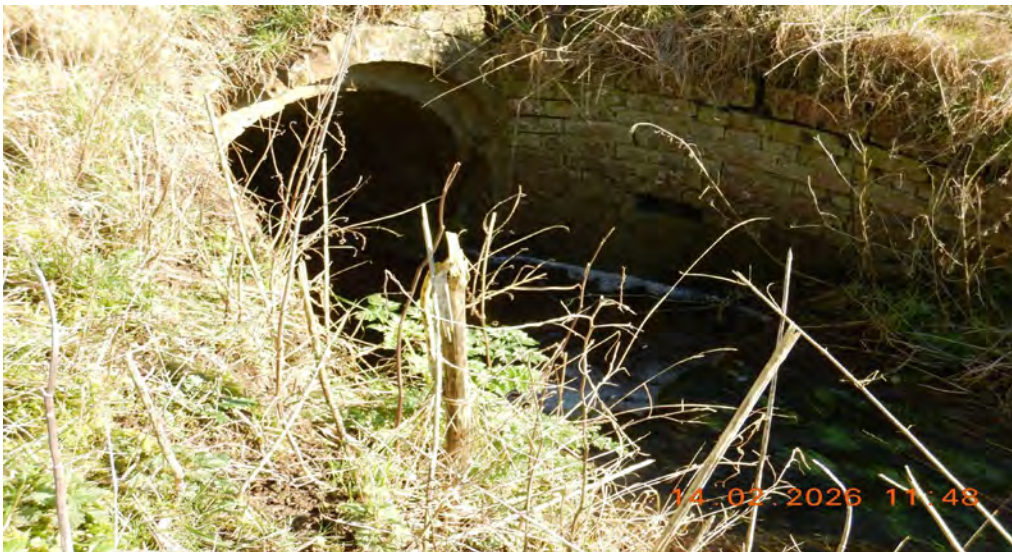
Figure 8.8 Showing Size of the Stream in the West of Site 5 as it flows under the B1527 (16th Century Brick culvert) and the North Boundary
