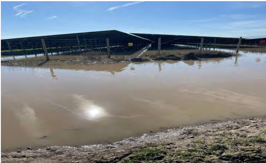
Figure 9.8 Photo of flooding at Cleve Hill Solar Park, North Kent on 2nd March 2026
