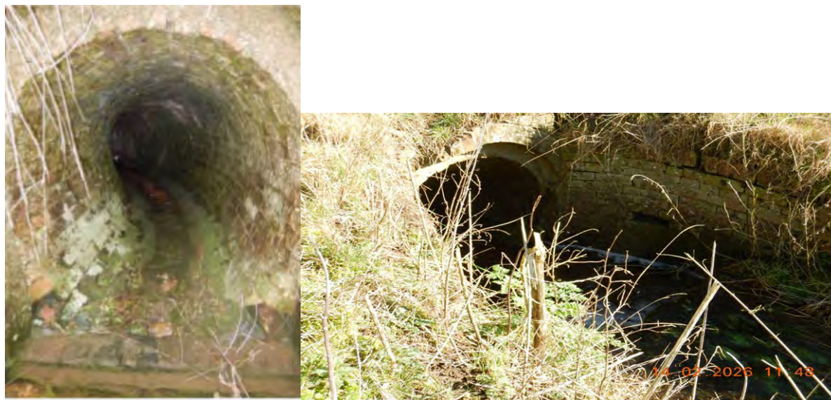
Figure 3.7 16th Century Brick culvert entrance situated in Site 5 running under B1527 to river Tas.
