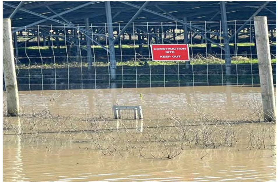
Figure 9.9 Photo of flooding at Cleve Hill Solar Park, North Kent on 2nd March 2026
