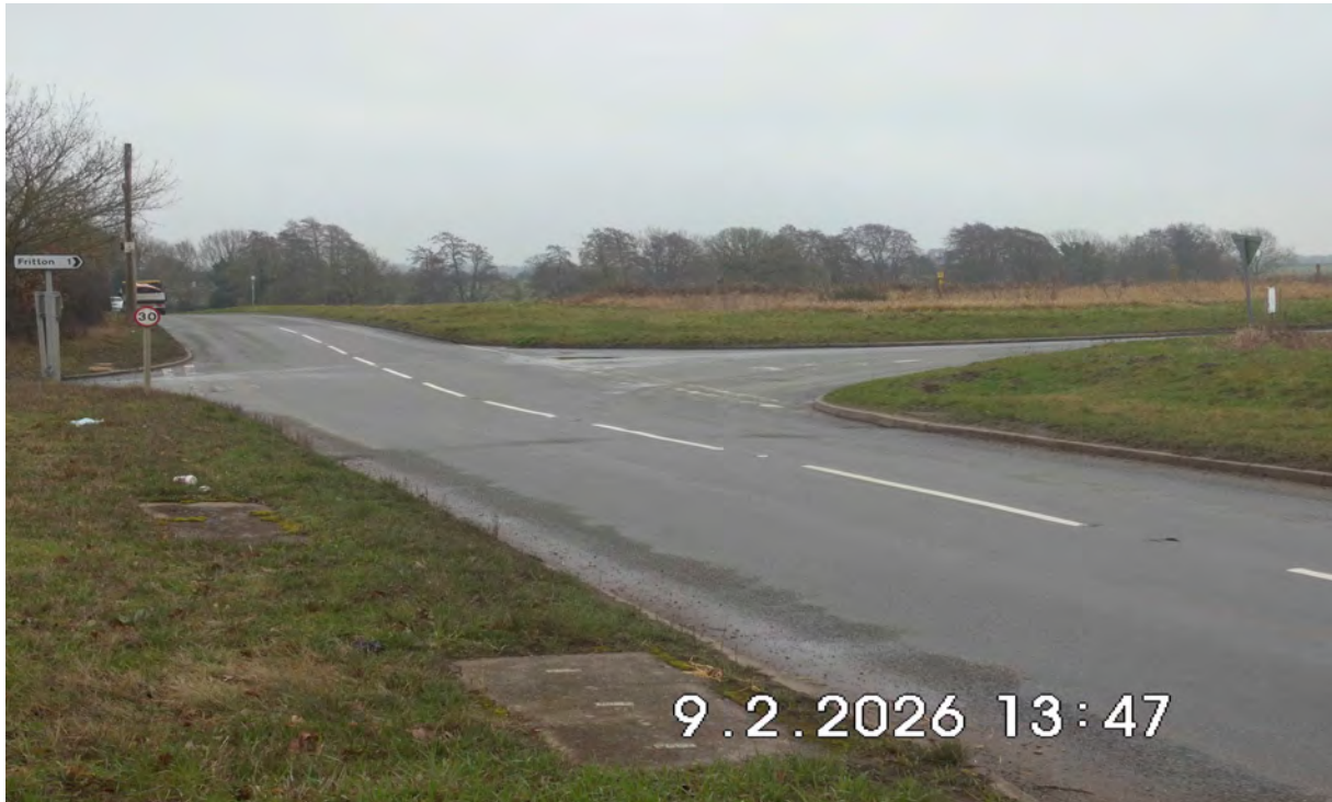
Figure 11.11 Photo of Junction of B1527, The Street and The Krons - easterly view. Vehicles from The Street (right side) National Speed limit just before the crossroads.
