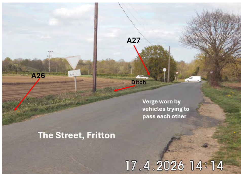
Figure 11.10 Photograph showing positions of proposed access points into Site 5 (A26) and into CRC7 (A27) in relation to the crossroads. Verge erosion due to the road being too narrow for large vehicles clearly visible on the right hand side.
